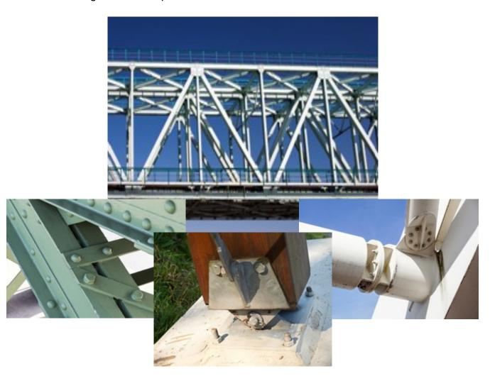
Some members will be in compression while others are in tension. Some are zero force members, with no internal forces at all, used to increase the stability and rigidity of the structure.
